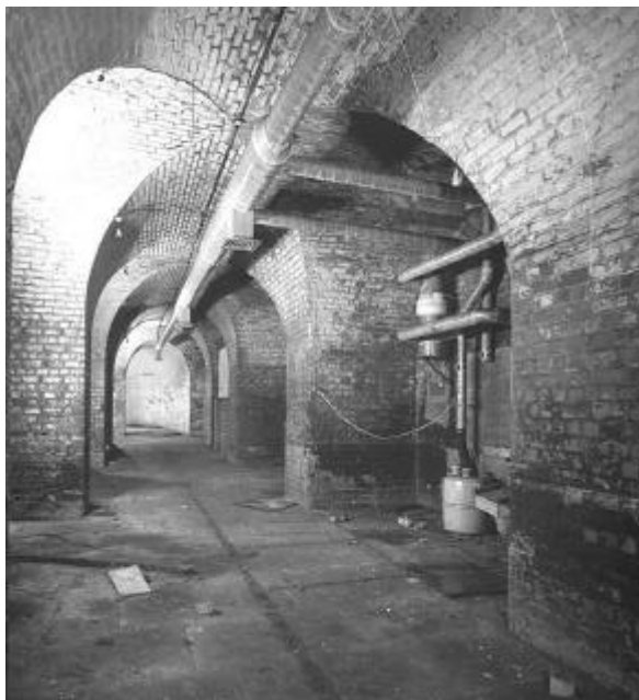
The south west caponier which housed the control room. Note the ventilation plant on the right
